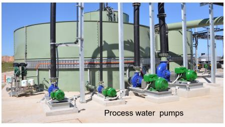
Doyle Pump & Engineering were engaged to work in collaboration with specialist industry consultant in the design and supply of purpose fit pump sets for a new sand washing/quarrying plant. As part of the design specification, Doyle Pump & Engineering provided a complete hydraulic and engineering design with detailed pipe sizing, technical data, CAD drawings and pumping solutions to meet specific end user requirements.
